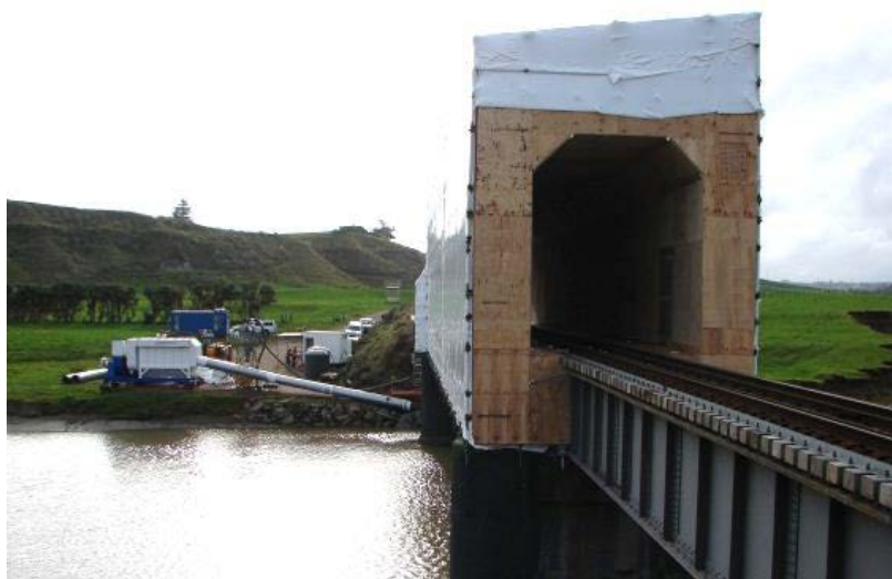
Figure 5.5: Full containment for repainting the Patea Rail Bridge (Supplied by TBS-Farnsworth)
