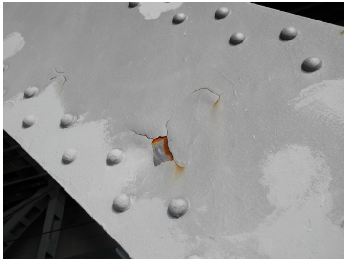
Figure 5.4: Example of damaged coatings – Auckland Harbour Bridge
