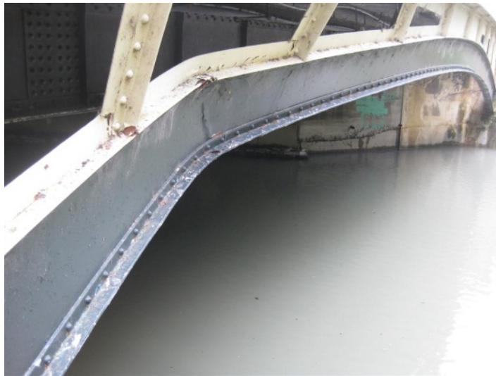
Figure 5.4: Example of damaged coatings – Auckland Harbour Bridge
