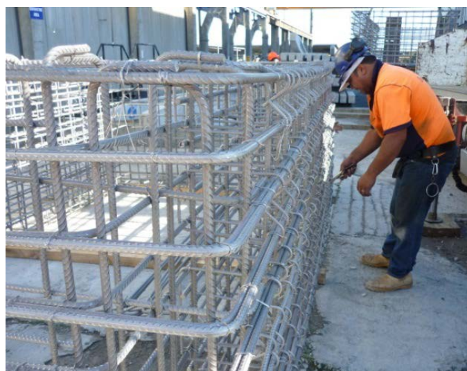
Figure 9.1: Wellington Harbour Culvert stainless steel reinforcement cage
